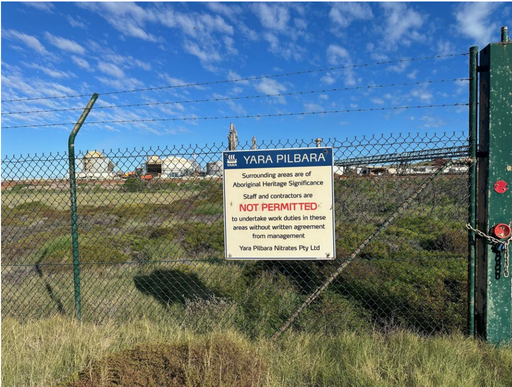
Condition 8: 2.5 m chain link perimeter fence and signage near western perimeter emergency exit (south side)
